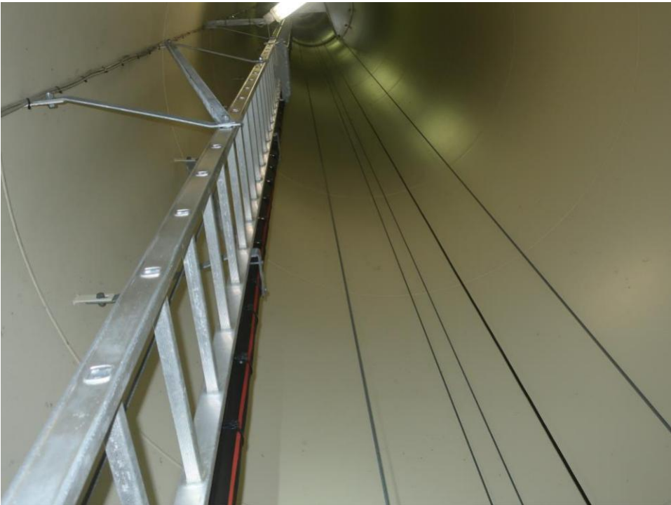
Overview inside tower
