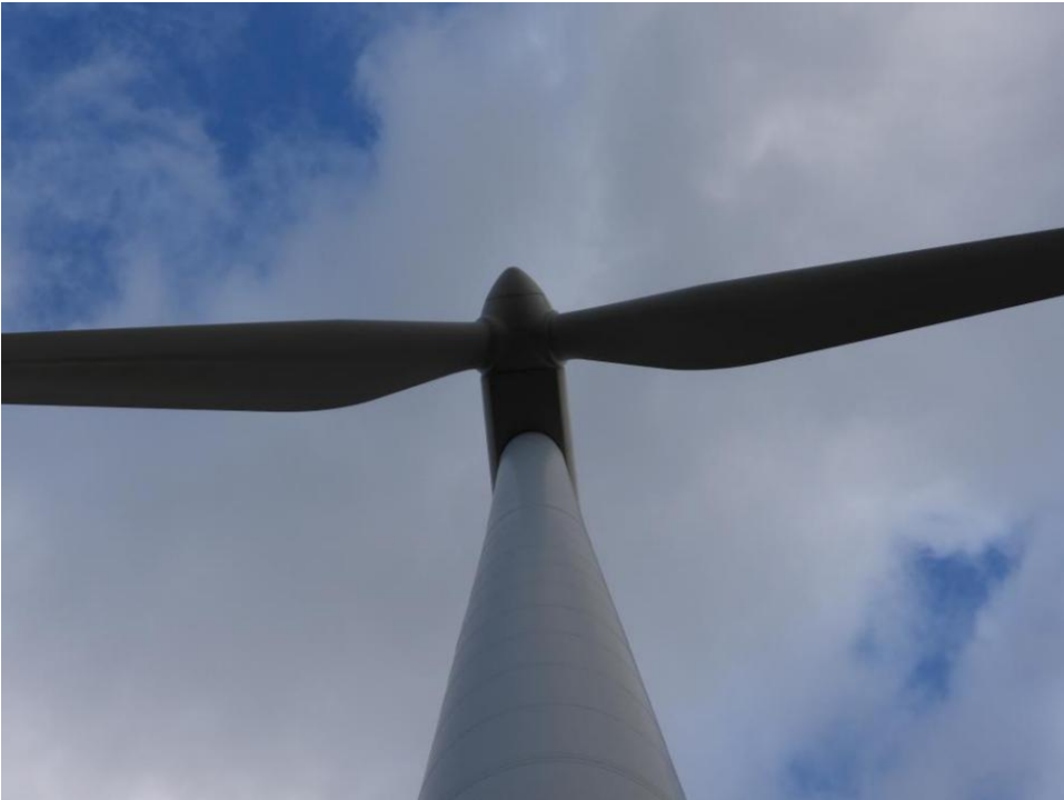
Overview nacelle and tower outside
