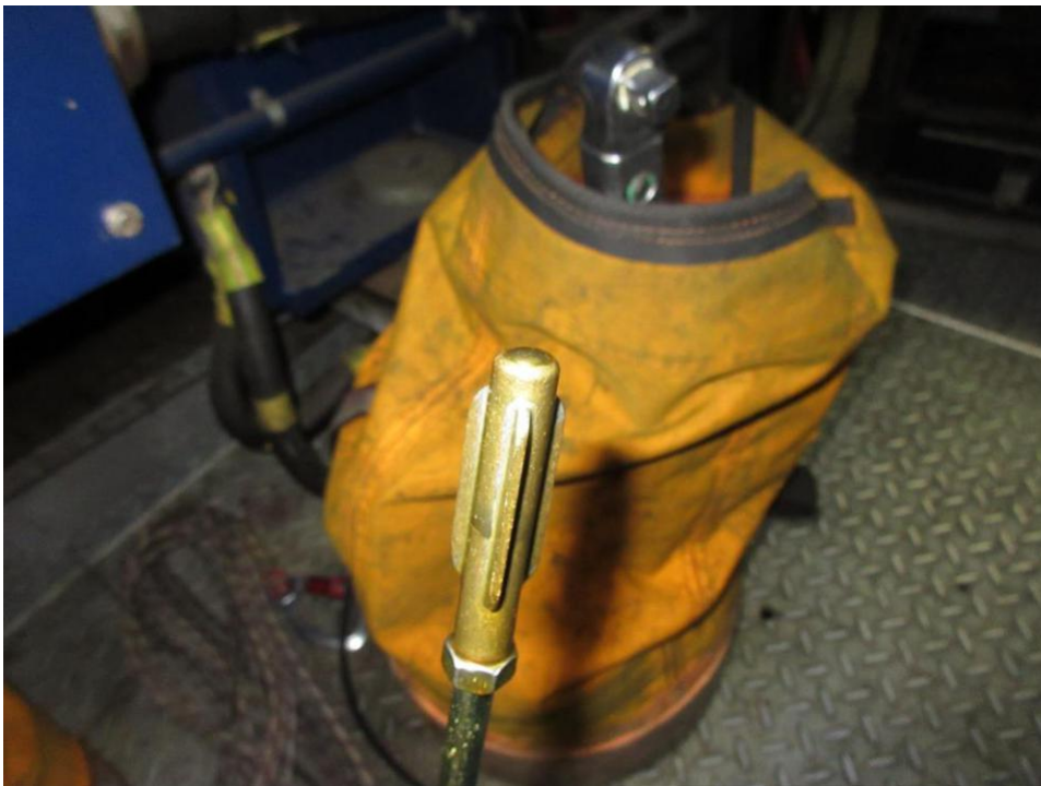
The magnet of the gearbox shows no irregularities.
